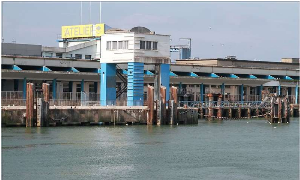
Figure 0.10 Boulogne kittiwake tower on old ferry terminal. Photo copyright J-M Sauvage.
