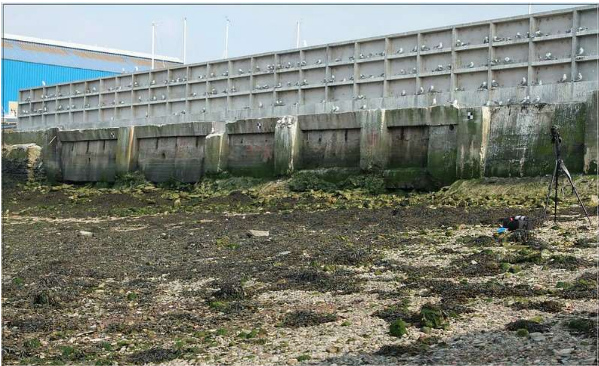
Figure 0.6. Boulogne-Sur Mer wall. Photo copyright J. M. Sauvage.
